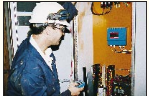
Infra-red hand held programmer used with wall mount version.
