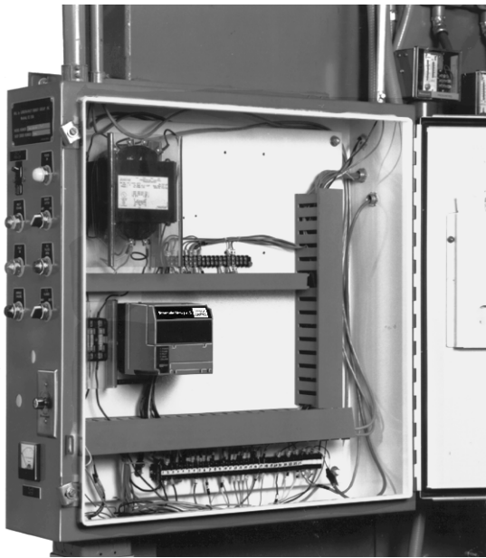
Fig. 7. Electrical panel installation.
