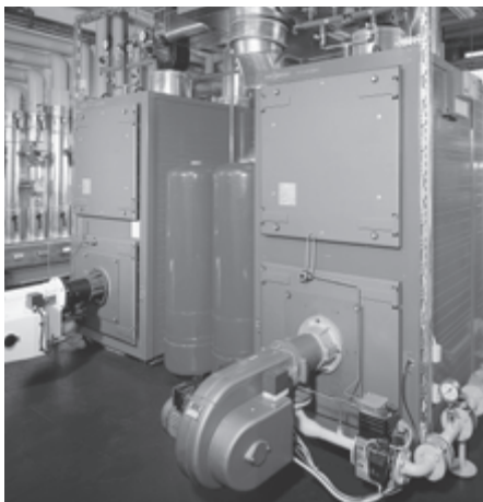
Gas inlet pressure monitoring on high-performance boilers
